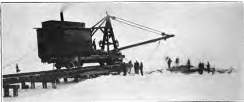
(e) Derrick Car at Work Clearing Intake Shaft at the Champion Copper Company Mill, January 17th, 1911.
